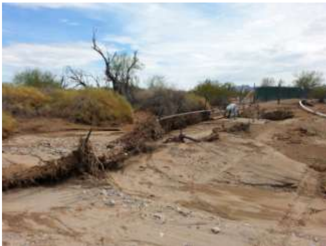
Storm Damage, July 2014
