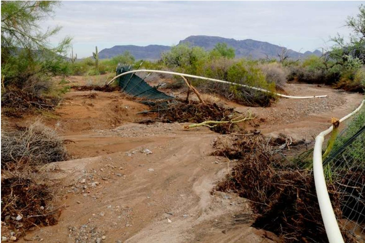
Damage along the midline fence, showing debris, missing fence, and broken irrigation pipe.
